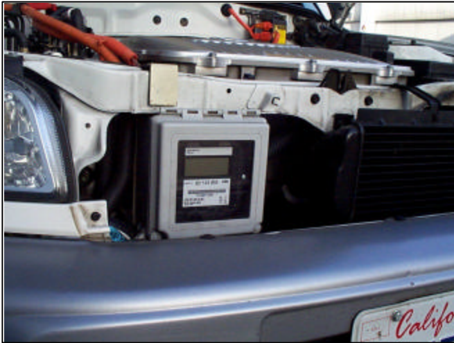
Figure 2. ABB kilowatt meter installed on a RAV4. It is located on the front of the passenger side of the RAV4.
